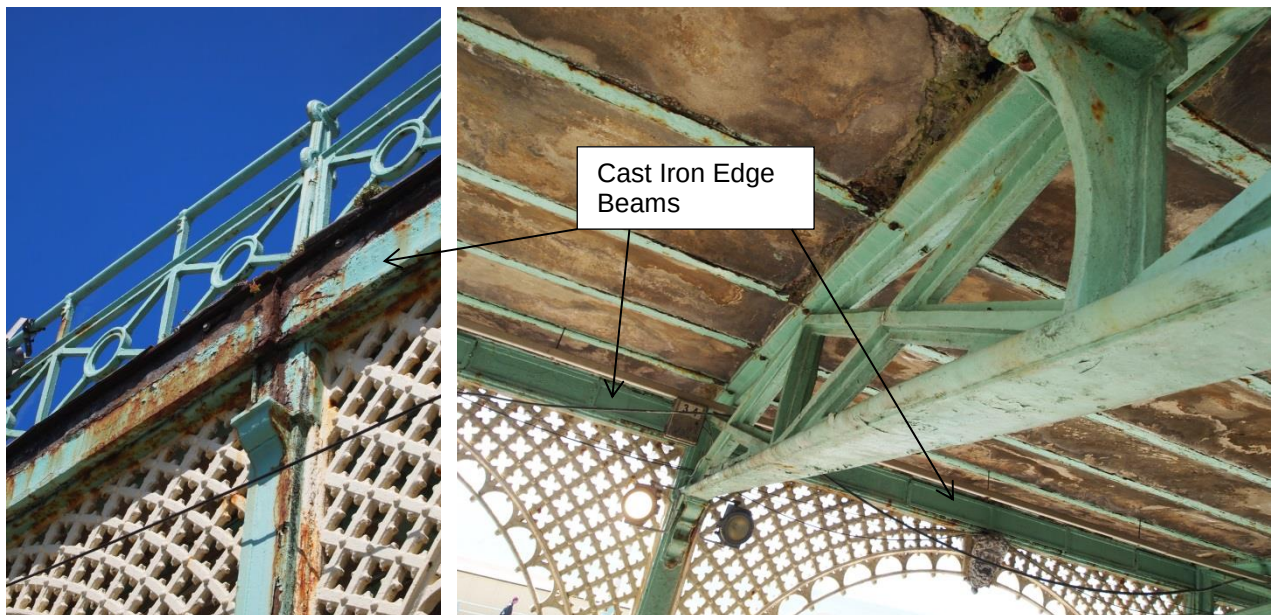
Figure 4.7 – Cast iron edge beam
