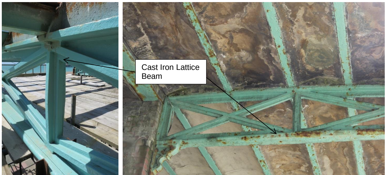
Figure 4.5 – Cast iron lattice beams
