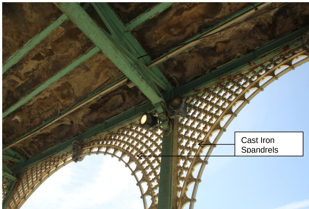
Figure 4.11 – Cast iron spandrels
