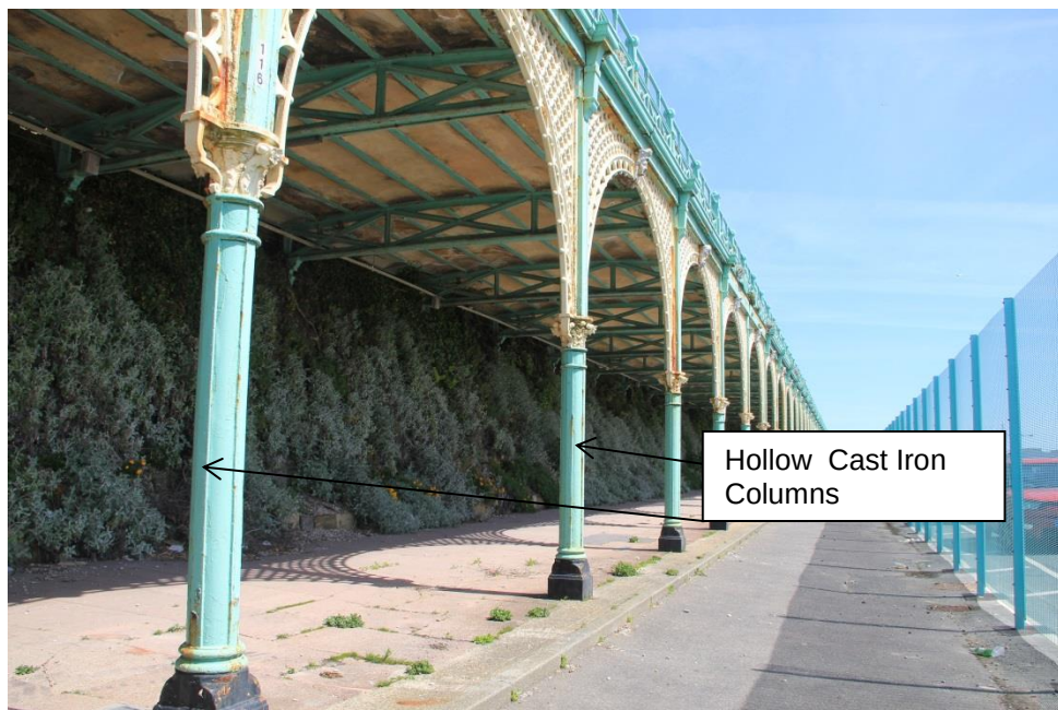
Figure 4.12 – Cast iron columns
